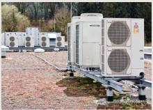
The installation of the VRF-R2 heat pump system with heat recovery strongly contributed to the DGNB certificate.
