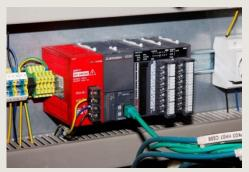
A FAG SmartController in the form of a Mitsubishi Electric PLC from the MELSEC L-series operates as a bidirectional gateway between the customer controller and sensors in the condition monitoring system. [Source: Mitsubishi Electric Europe B.V.]
